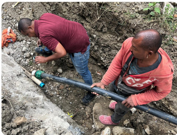
Community members are working to bring water to nearby communities
